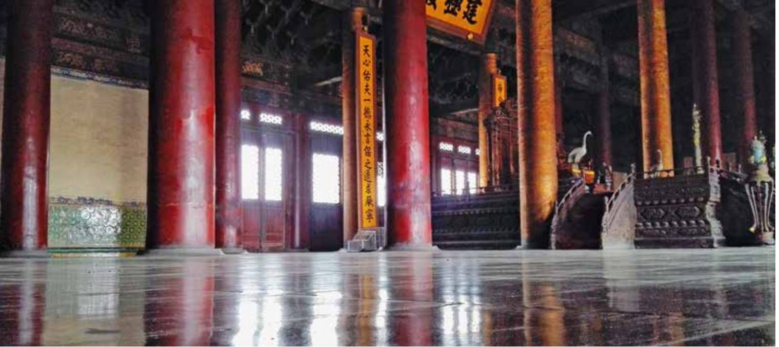
Forbidden City in Beijing, floor made of Lumu bricks (photo: Tan Hongyu)
